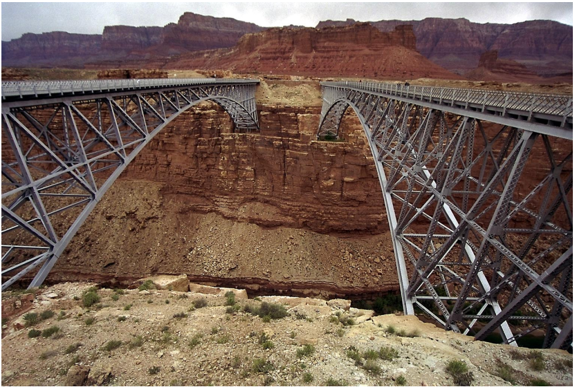
Arizona's Historic Navajo Bridge spans Marble Canyon in a graceful silvery arch approximately 470 ft. above the Colorado River. The original 1928 bridge that replaced Lee's Ferry is on the right. The newer, wider bridge on the left was completed in 1995. Photo Paul Fretheim
